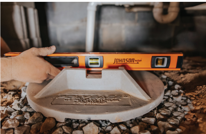
PolyBase® installed on 57 stone.
