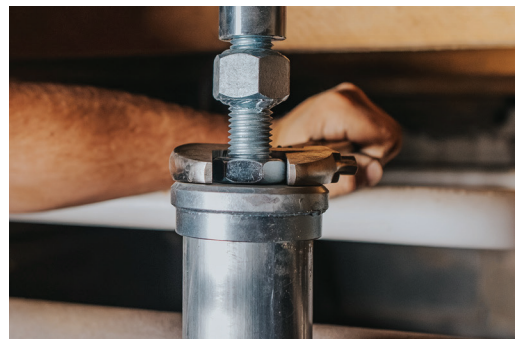
Tightening adjusting jam nut.
