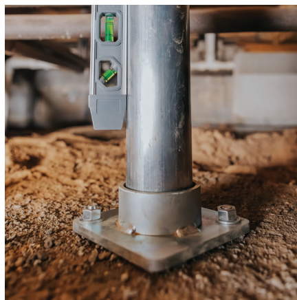
Base Mount installed on concrete footer.
