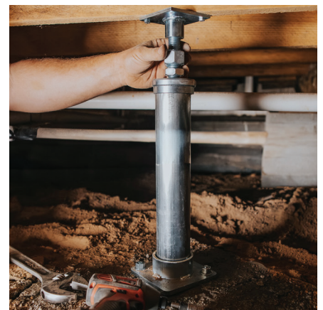
Assembled system on concrete footer.
