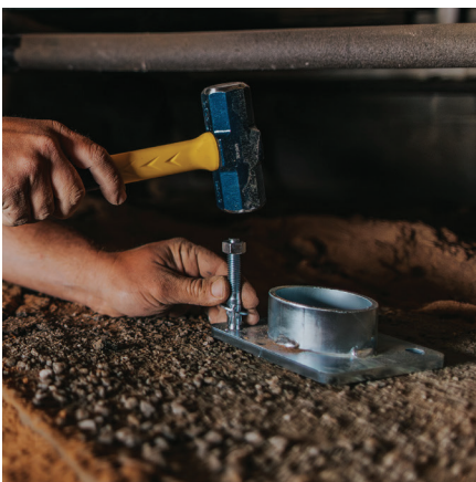
Anchor bolts installed into concrete footer.
